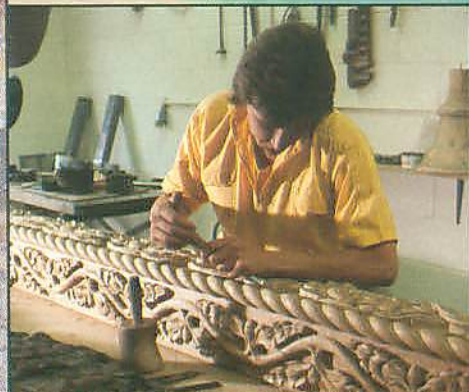
Restoration work at Little Moreton Hall, page 16
