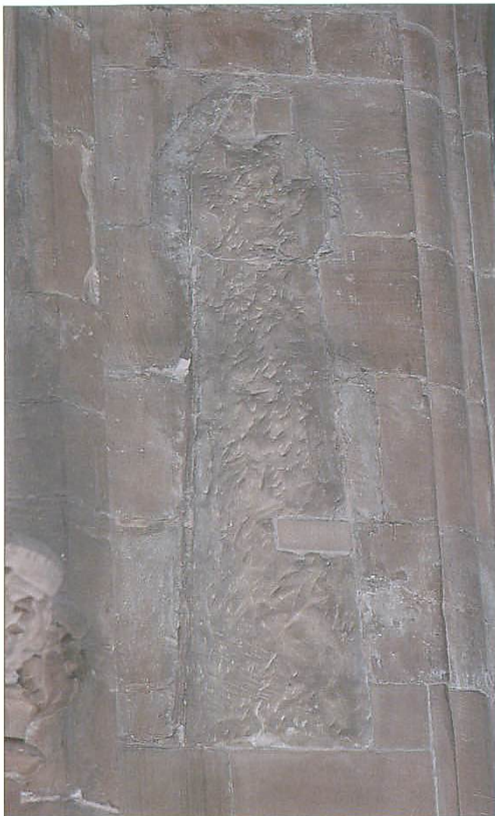
The 'cross shaft' in the east wall of the south transept
