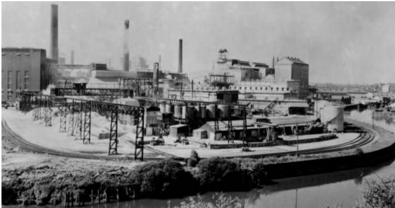
Left: Alkali works, Winnington. Above: Widnes chemical industry.
