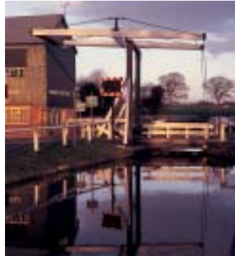
Wooden lifting bridge over the Shropshire Union Canal. Built in 1790 by Thomas Telford.
