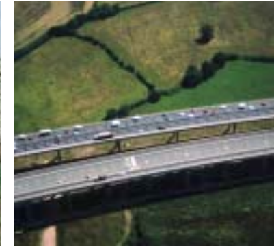
The Thelwall Viaduct carries Britain's longest motorway, the M6 across the Manchester Ship Canal and River Mersey. It was opened in 1963.
