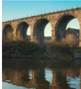
Railway viaduct for the Northwich – Chester Railway, opened in 1869. It crosses the rivers Dane, Weaver and the Weaver Navigation. It has fifty arches and is 950 metres long.
