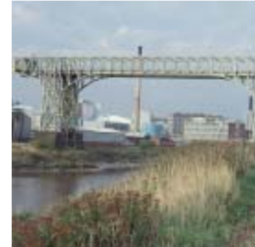
Transporter bridge built between 1913-15, to link Crossfields soap works on both sides of the river at Warrington Bank Quay. It could transport trains as well as road vehicles and pedestrians. It has not been used since the 1950s.
