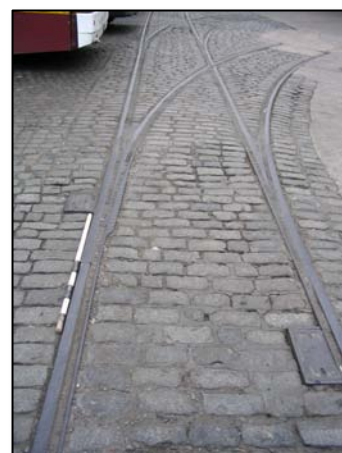
Figure 5: Early 20 th century tramlines still surviving in the modern street surface (Castlering Archaeology)
