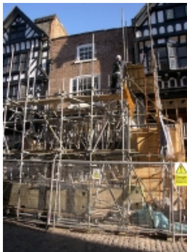
Repairs in progress at 8–10 Northgate Row
